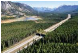
A wildlife crossing spans the Trans Canada Highway in Banff National Park in Alberta, Canada. A similar crossing might be in store for Interstate 70 over Vail Pass. ( Tony Clevenger, WTI )
