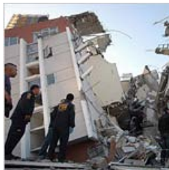
Stress of Sliding Plates Builds Near Chile
