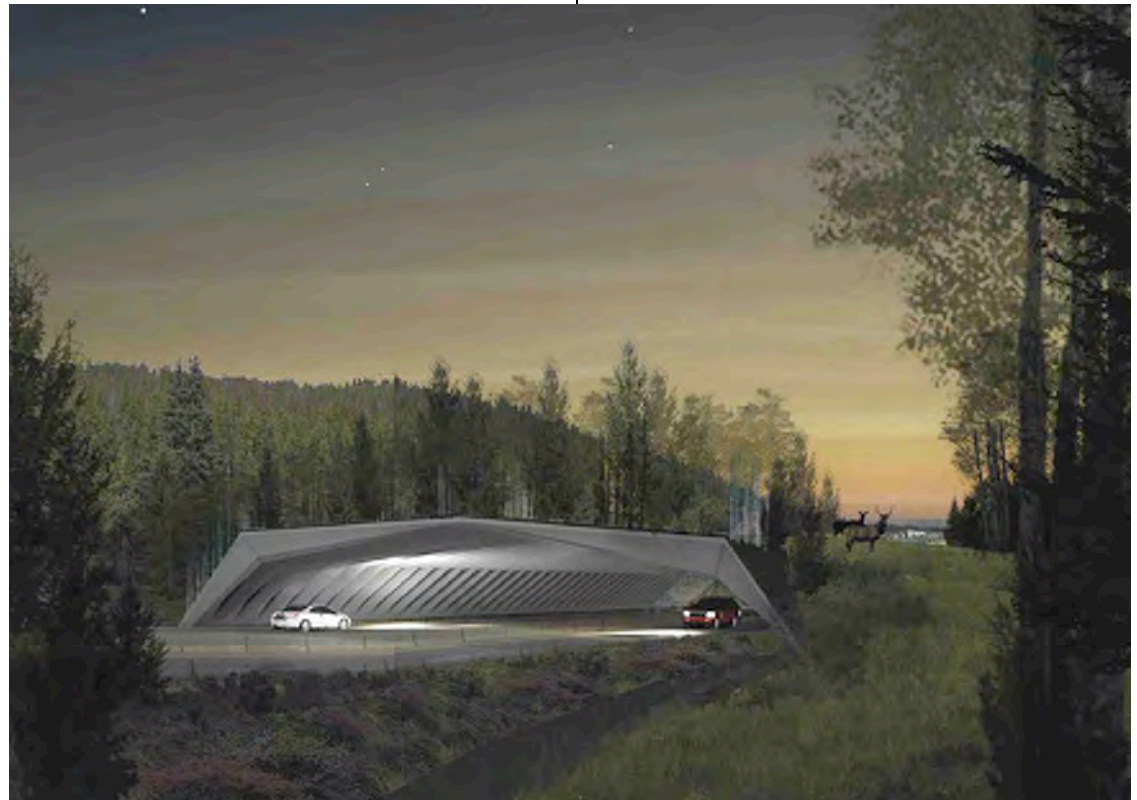
Building elements called hyper vault modules are at the core of the winning entry, shown here as how it might cover the lanes of I-70, the potential for a train of some sort, plus the existing bicycle path.
