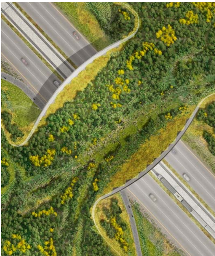
Click above image to view slideshow The Olin Studio with Explorations Architecture (Paris), Buro Haphold (London) and Applied Ecological Services
